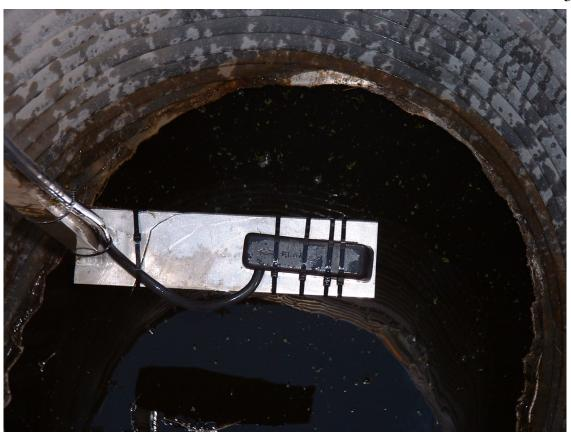
g. Area-velocity Probe Attached to Mounting Pole
