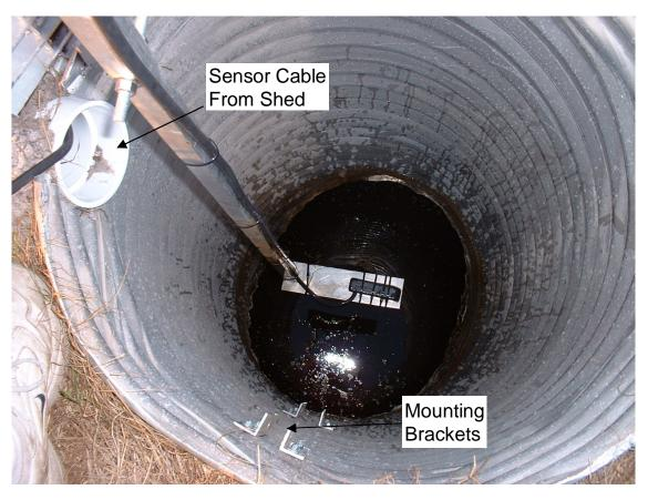
h. Riser Structure Used for Installation of Flow Probes
