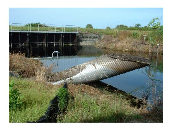
Figure 5-1. Dislodged Intake Pipe.
