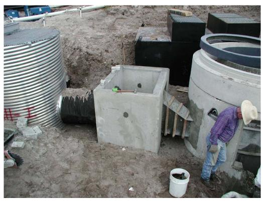
1. Connection Structure for CDS Unit
