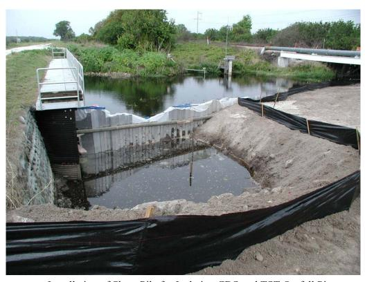
n. Installation of Sheet Pile for Isolating CDS and TST Outfall Pipes
