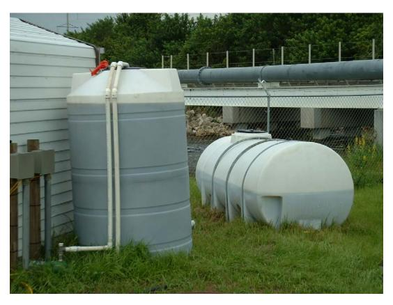
Figure 6-2. Storage Tanks for Alum and Polymer.
